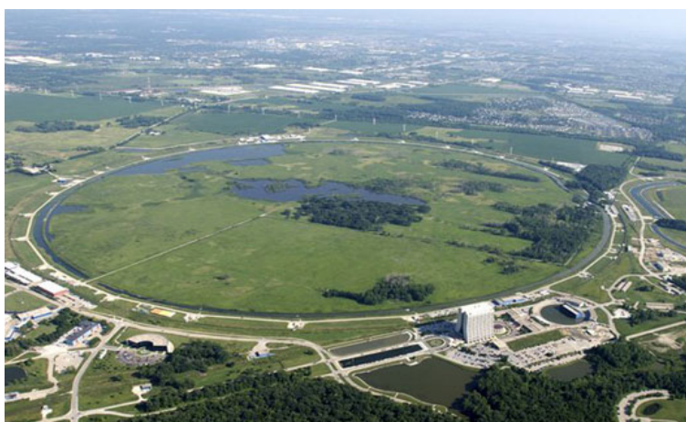
Figure 2.3: The aerial view of the Tevatron accelerator.
